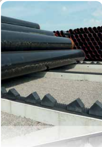
Pipe Stop on concrete beams
